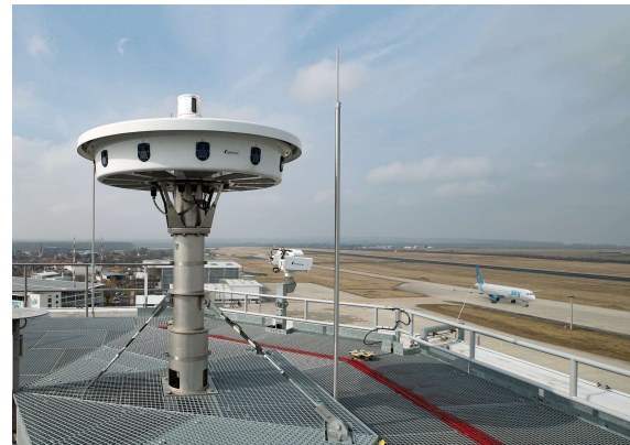
Figura 2: Torre de control remota (alt.) [3]
