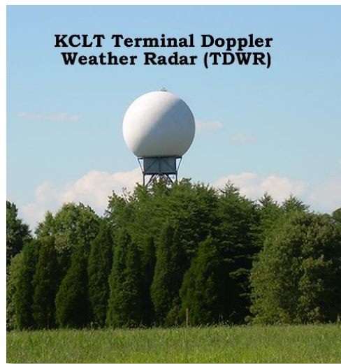
Figura 9 - Radar Doppler de Terminal (TDWR) - CLT
